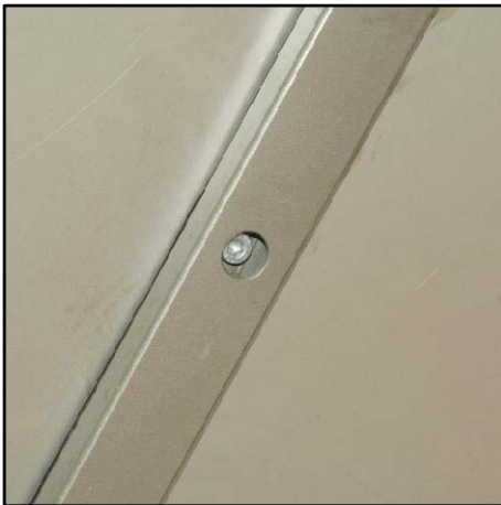
5 roof metal/roof props inside
